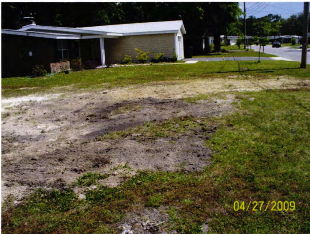
Picture 2: 295 Birch Dr. excavation site.
